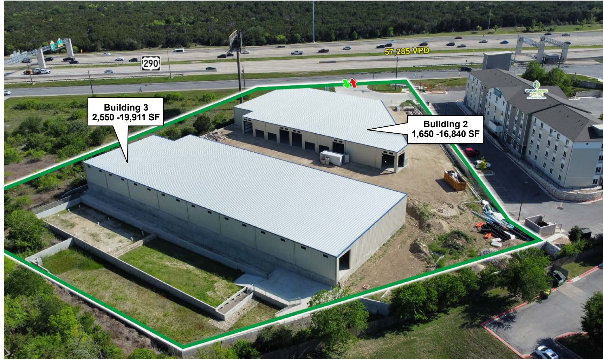
Construction Progression April 2025
